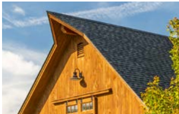
Cantilever Ridge Beam with Cow Catcher Peak
