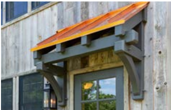
Timber Frame Eyebrow Roof Above Entry Door
