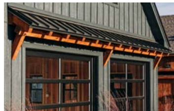
Modern Timber Frame Eyebrow Roof
