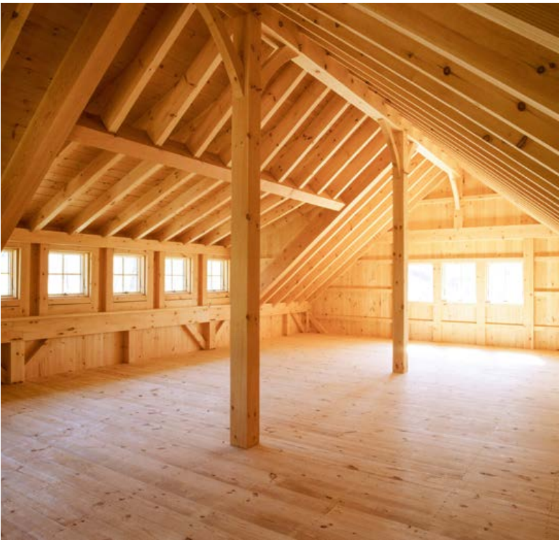
SIP Installation Process
