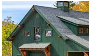
Timber Overhang Corbels
