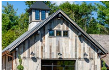
Timber Show Rafter with Corbels
