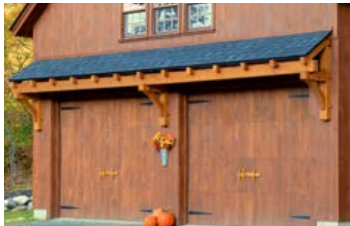
Timber Frame Eyebrow Roof Above Overhead Door
