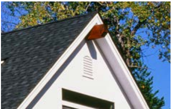
Cantilever Ridge Beam
