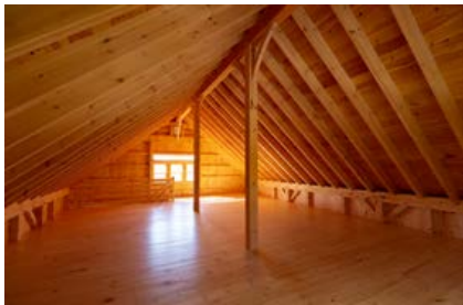
Rafter & Structural Ridge Beam
