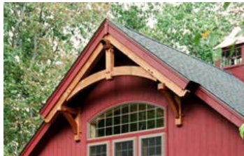
Turkey Tail Peak with Timber Truss
