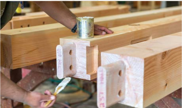
Applying Wax End Sealer to Joinery
