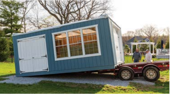
Step 2: Building Placed on Stone Pad
