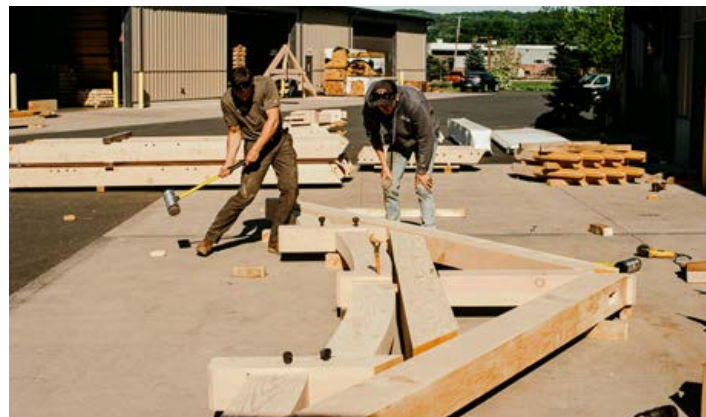
Timber Truss Assembly
