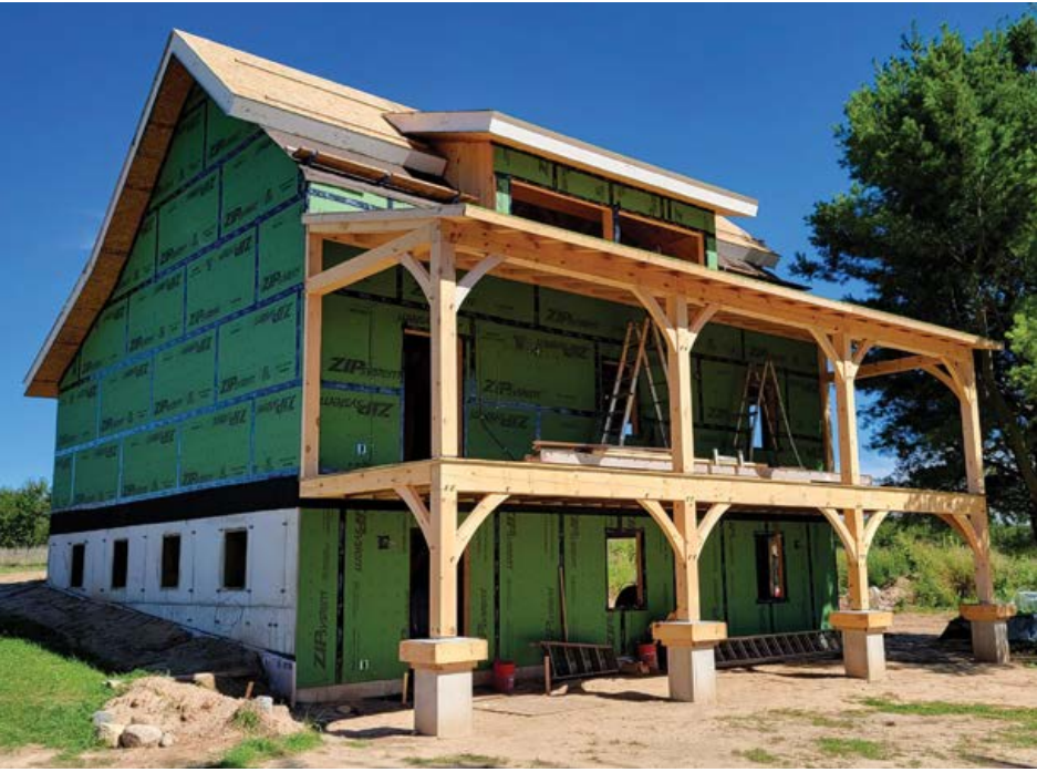
ZIP R-Sheathing Shown on Walls; 8.25" SIPs Shown on Roof
