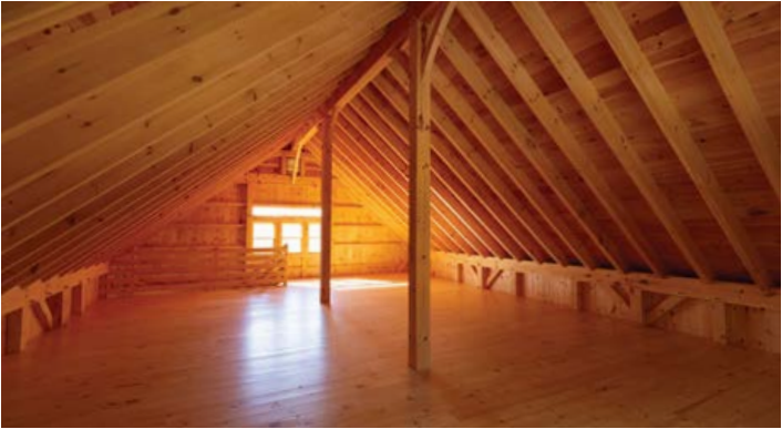
Rafter & Structural Ridge Beam
