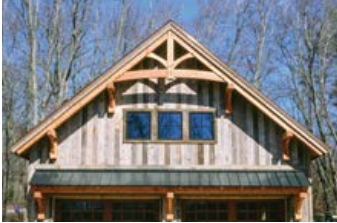
2' Gable Overhang with Timber Truss Accent & Show Rafter
