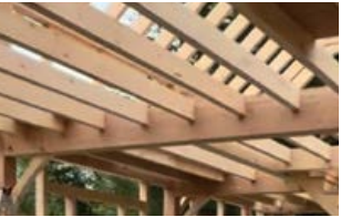
Solid Sawn Douglas Fir Beam
