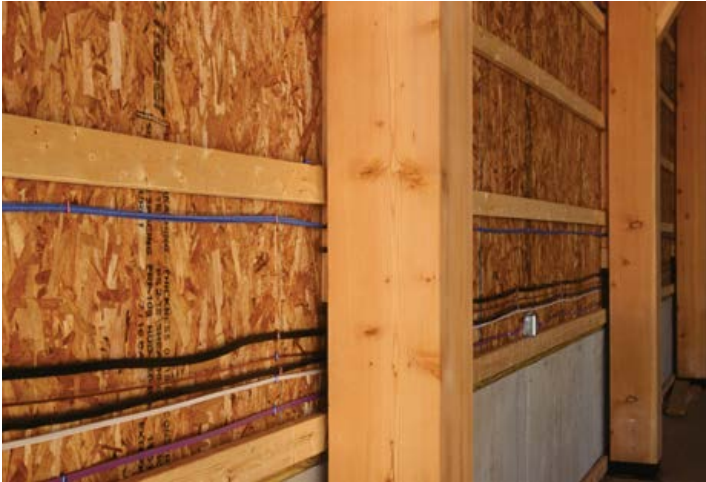
Spacers Create Room Between SIPs and Timbers for Utilities
