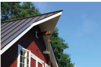
Cantilever Ridge Beam with Cow Catcher Peak
