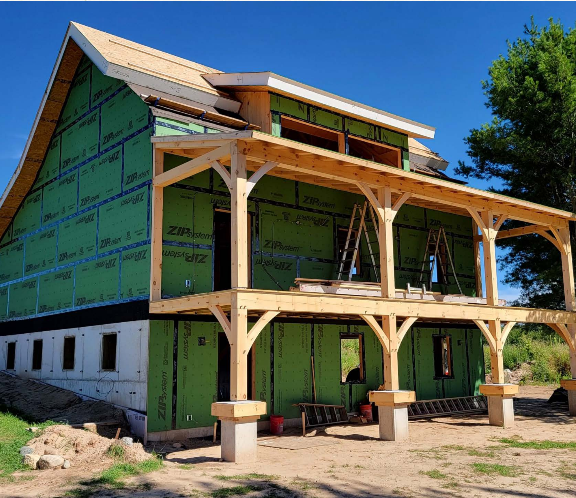
Zip-R Sheathing Shown on the Walls, and 8.25" SIPs Shown on the Roof.
