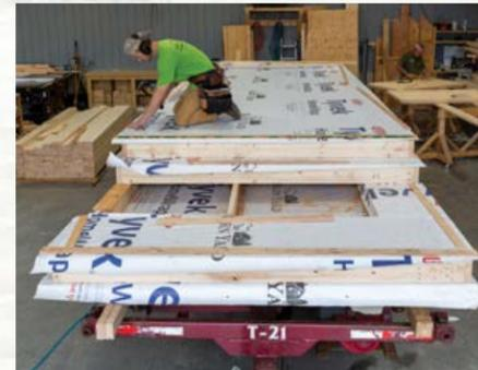
**Wall Construction.** We build the wall panels in a controlled environment to ensure the highest quality.
